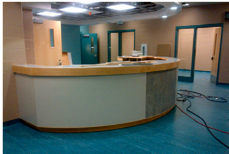
Under construction: Northeast Nova Scotia Correctional Facility
